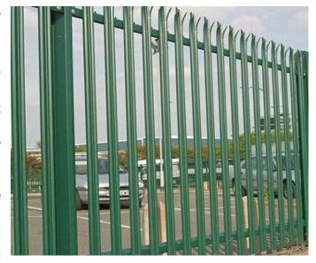
around many industrial sites. Palisade is more secure than many other fencing systems so wherever security is priority palisade is used.
